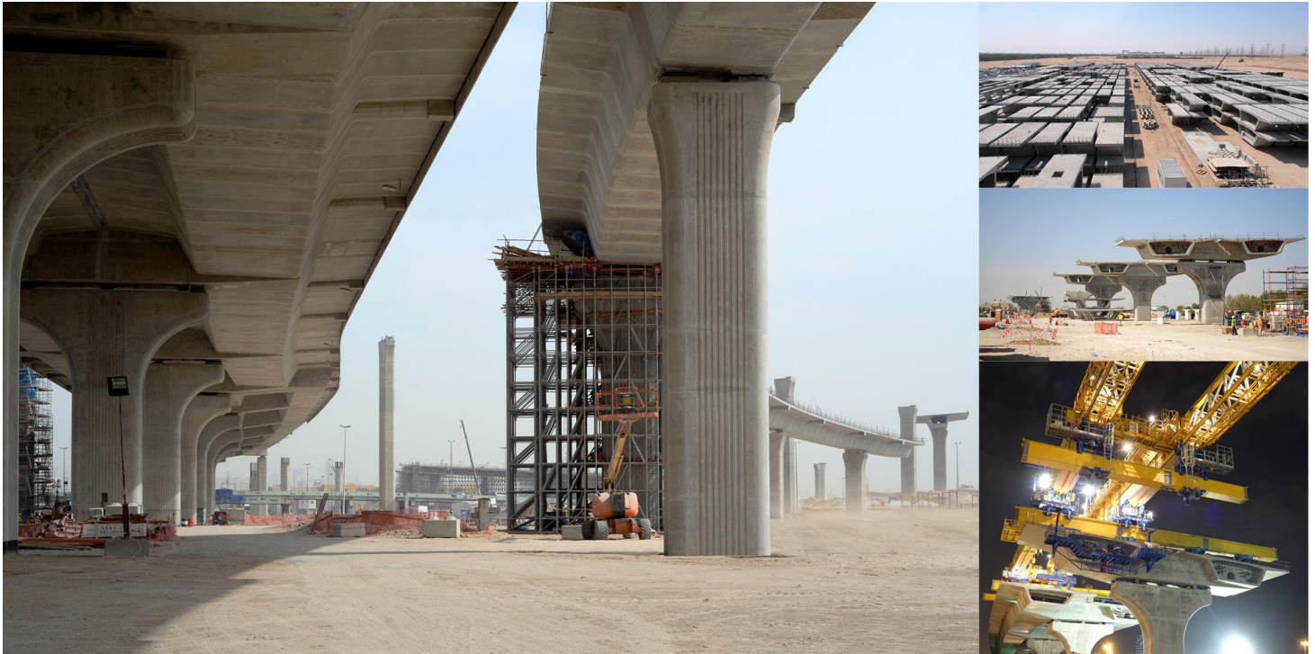
continuous viaducts with segmental construction overall length 11 km, typical span: 45.00 m.
